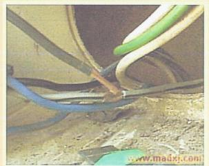
Push the copper strands of the gray (or brown) wire apart in the middle. Insert the bare end of the black wire in here.
